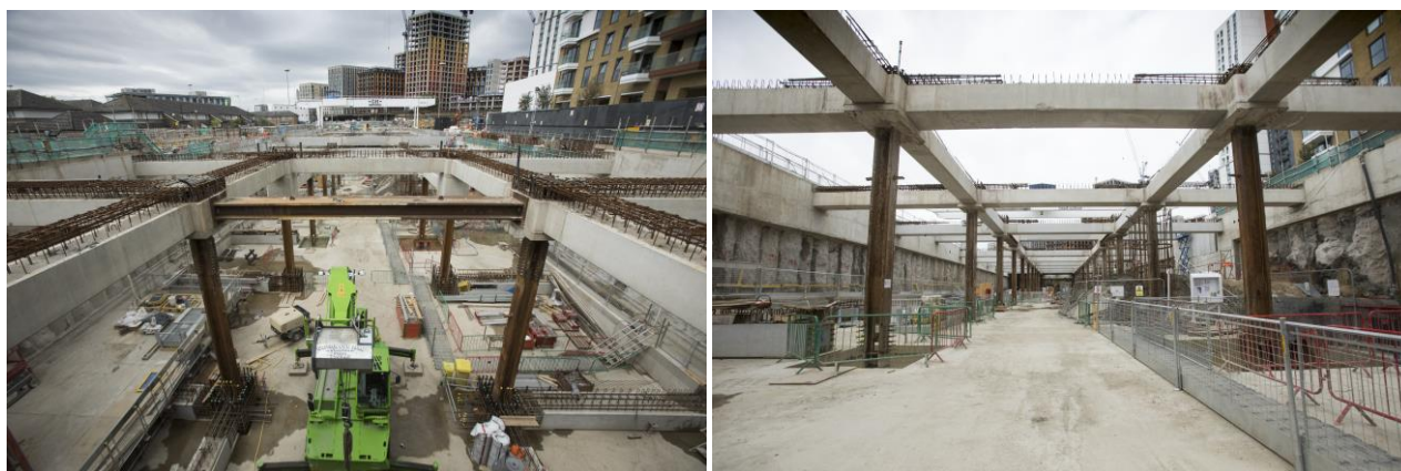
Above – the Nine Elms station box under construction.
