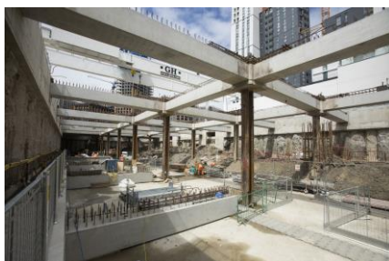
Above – installation of precast beams
